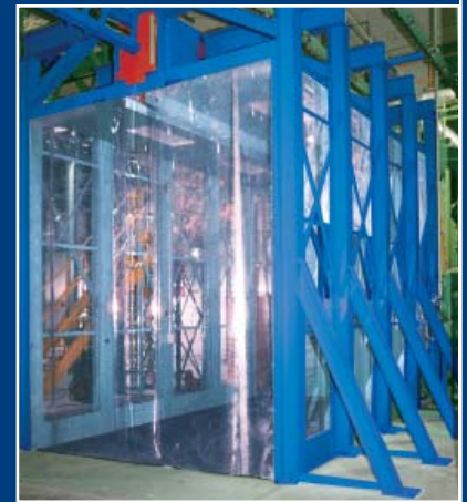
Lighted enclosure for abrasive removal
